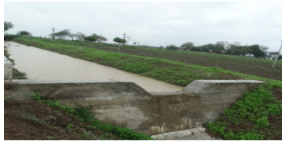
FIG : Cement nala bund
